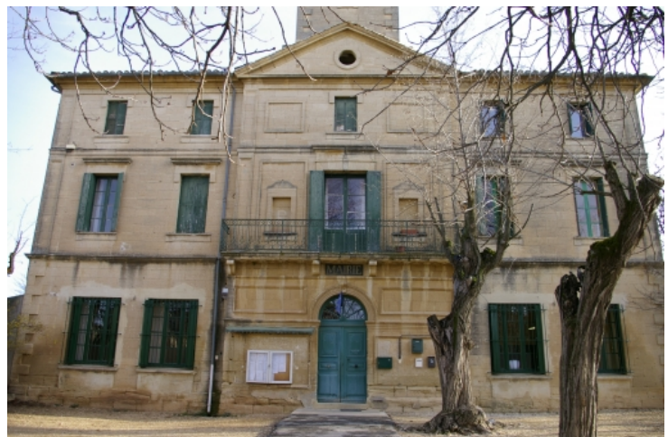
Façade principale, sud © Jennifer Gomez (2007).
